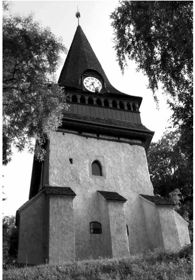
Fig. 2. Bell Tower built in 1554 (Photo: E. Gyulai)
